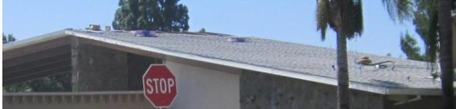
the office. A coat of weatherproof sealant was applied before the new shingles were laid on Thursday and Friday. Soon those new shingles will be hidden beneath an array of solar panels helping to generate 21<sup>st</sup> Century energy for our Recreational Complex. The roof over the Annex
